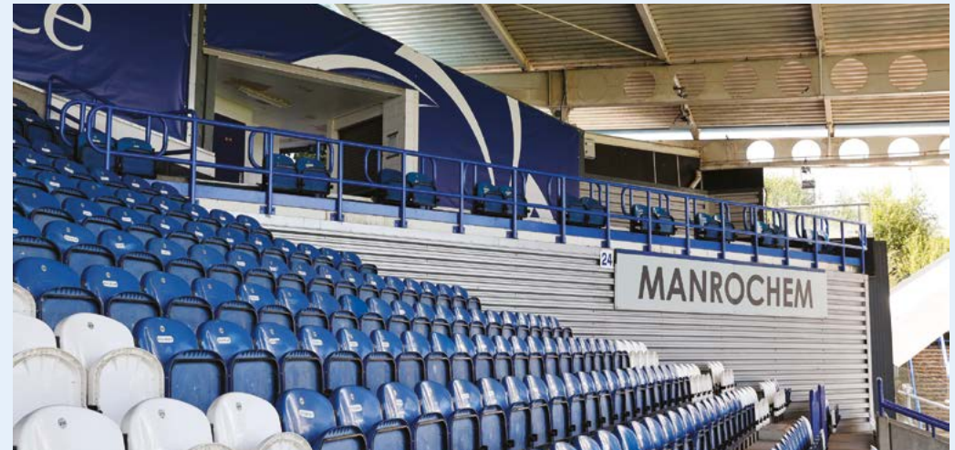
Figure 8 Raised platform for wheelchair users and their companions at the back of the Chadwick Lawrence Stand.
