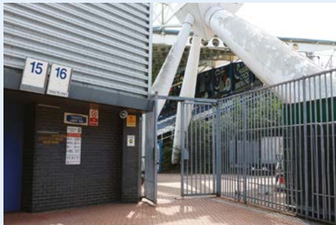
Figure 18 Accessible Entrance next to Turnstile 16
